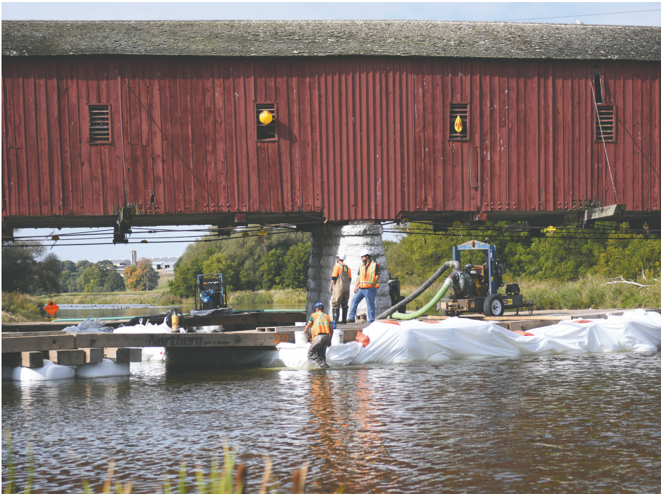
Workers have built a temporary span across the Grand River to help them restore the West Montrose Covered Bridge. Julian Gavaghan
